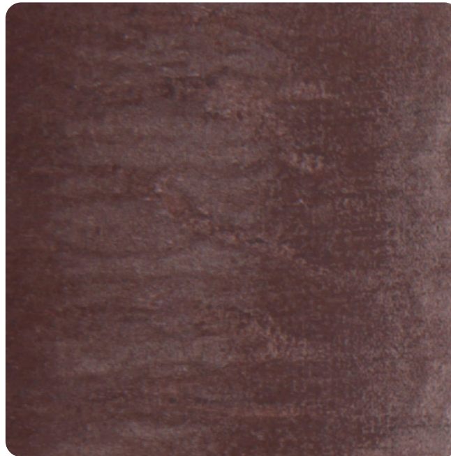
Temperature stains without integrity damage of laminated coating
